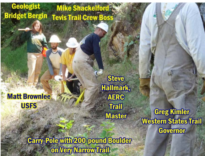
Belaying the boulder to the trail-bed
