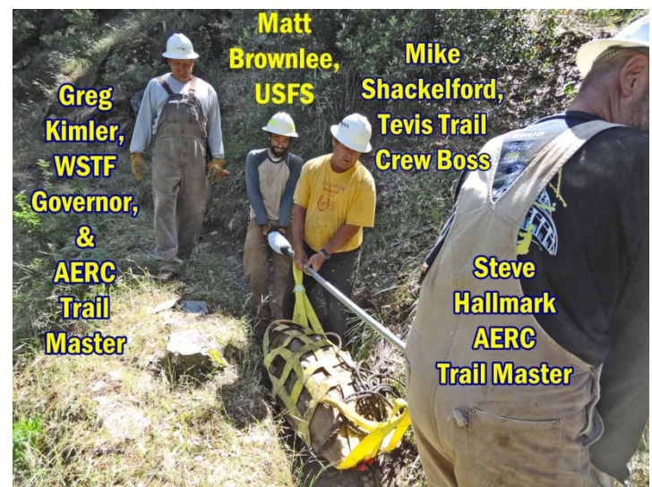
Belaying and lowering loose boulder in carry-sling
