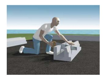
•All slabs to be nailed with the supplied special insulation nails. One in each corner of the slabs.
