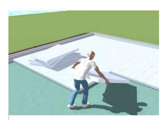
**7** • Cut the last element with a teflon coated handsaw.
