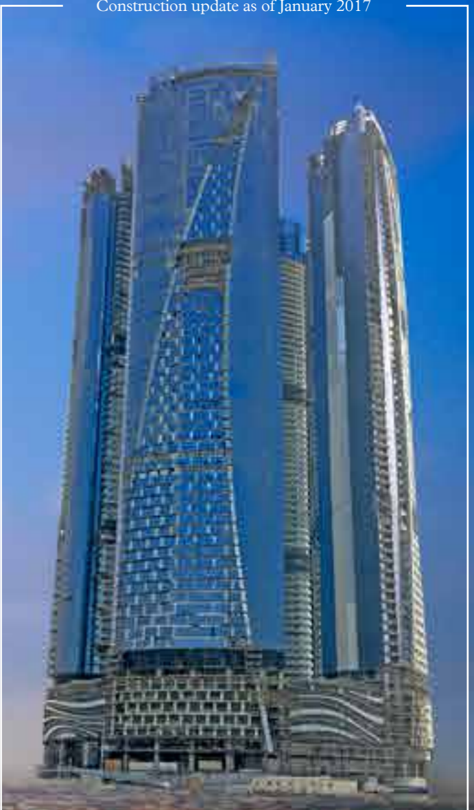
Construction update as of January 2017
