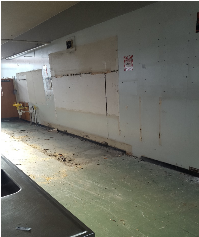
Level 1 and 2 strip out, before setting up enclosures, sealed areas with ACD contamination
