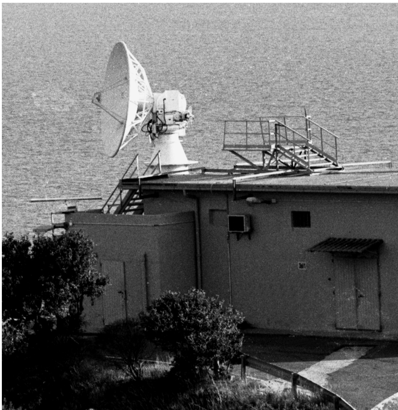
Fig 2 RIS-3C Tracking radar in the “ Torre Murtas ” station, the parabolic antenna reflector is visible
