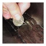
end on the ridge between passes. If you can fit the end of the paper clip through the gap, the ridge is too deep. Grind smooth and redo caps.
