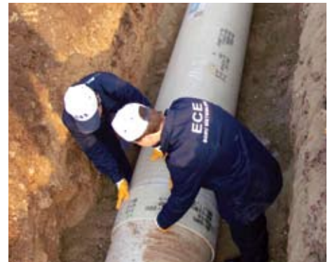
Granular materials are filled up to the 70% of pipe outside diameter then selected, native soil is compacted up to (h) distance. (h) distance is min. 100 mm max. 300 mm.
