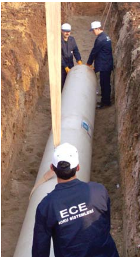
Granular materials are filled up to the 70% of pipe outside diameter then selected, native soil is compacted up to (h) distance. (h) distance is min. 100 mm max. 300 mm.
