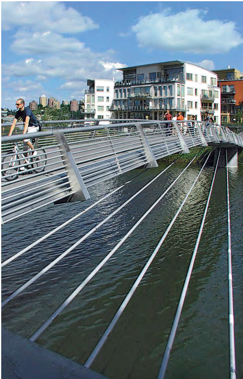
Duplex stainless steel bridge in Stockholm, Sweden (Source: Outokumpu)
