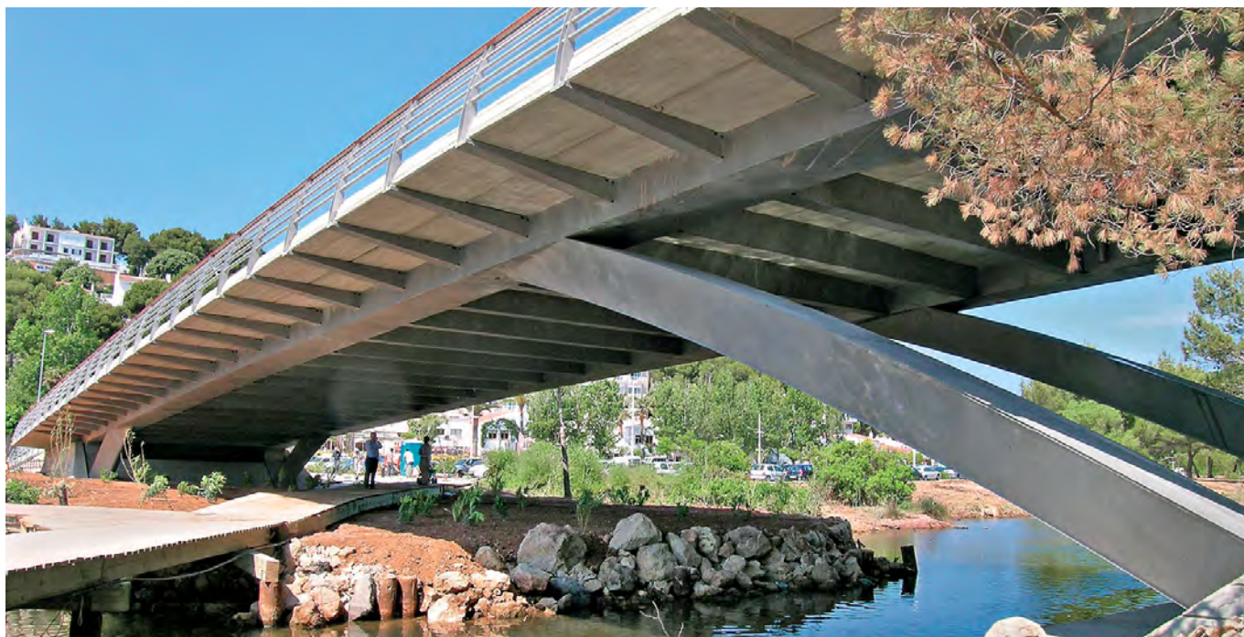
Bridge in Cala Galdana on Menorca fabricated using 2205 duplex stainless steel (Source: PEDELTA)
