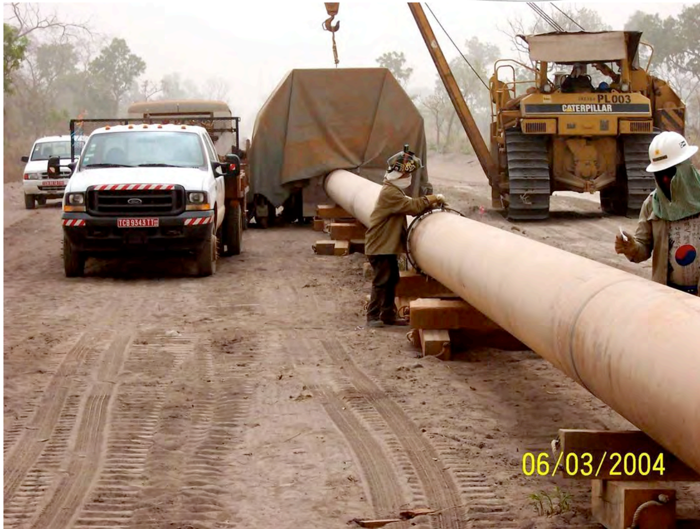
Chad - Double-Joining 24" O.D. X65
