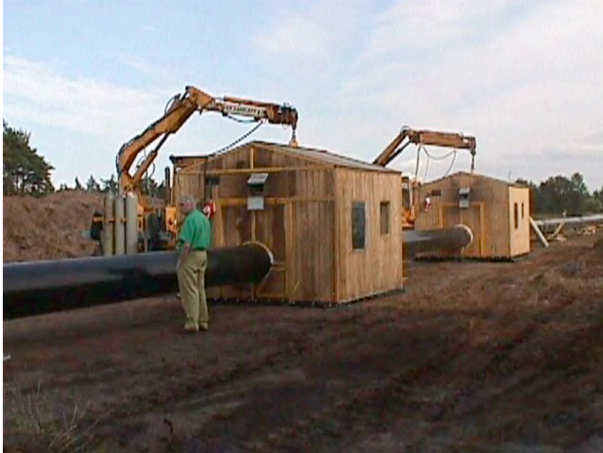
Dong Gas Pipeline, Denmark 24" x 15m wall, X-65 187 km Contractor: Per Aarsleff
