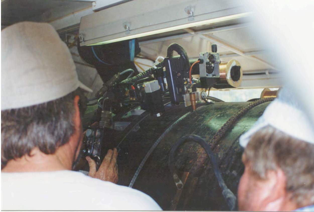
Otis Eastern Water Pipeline Project - 48"O.D.
