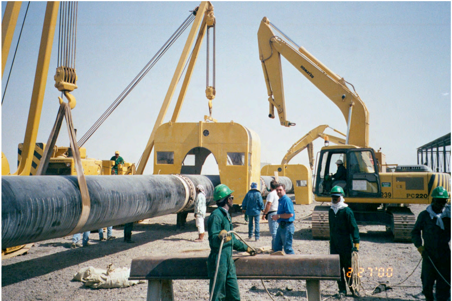
Hidd Bahrain Water Pipeline 42", 56", 72" O.D. x 15mm wall X60, 10 km
