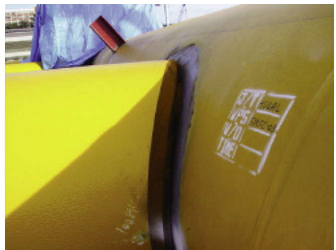
Fig. 3 — Fitup of a TYK field joint.
