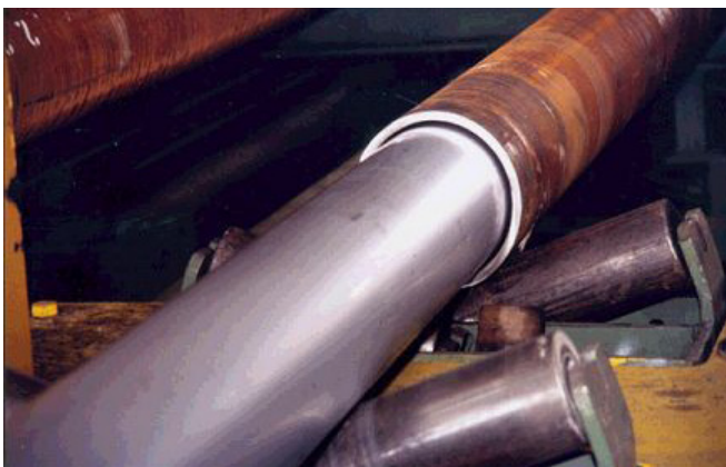
FIGURE 11. Telescopic alignment of liner and outer pipe prior to hydraulic expansion to form lined pipe.
