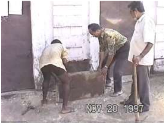
Removing the stone from wrongly inserted wall of the Chapel
