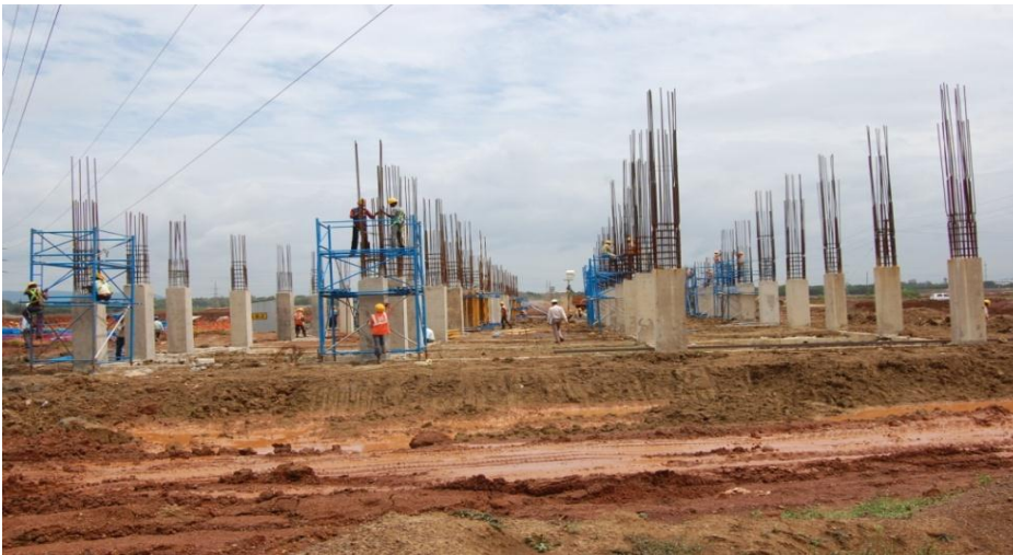
Civil work in progress in substation building in sinter plant
