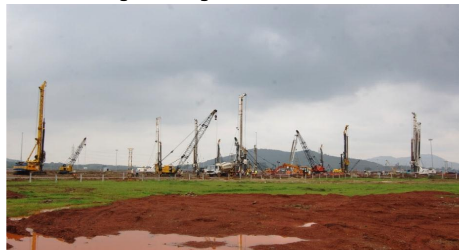
Piling work in SMS area in progress
