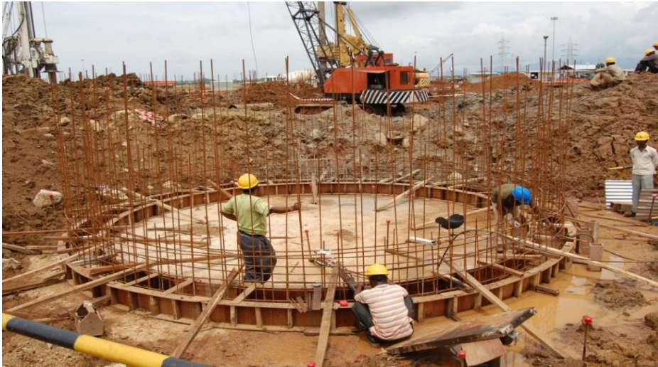
Civil works in progress in dedusting stack
