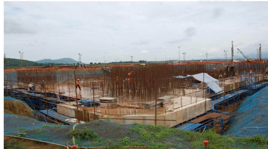
Casting of a single foundation of 5500 m3
