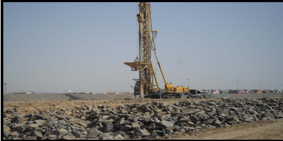
Stone columns work in progress
