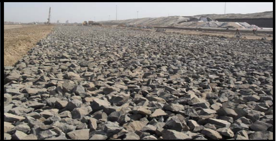
Preparation of ground for rail track in progress
