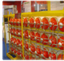
CNG Gas Storage Cascade
