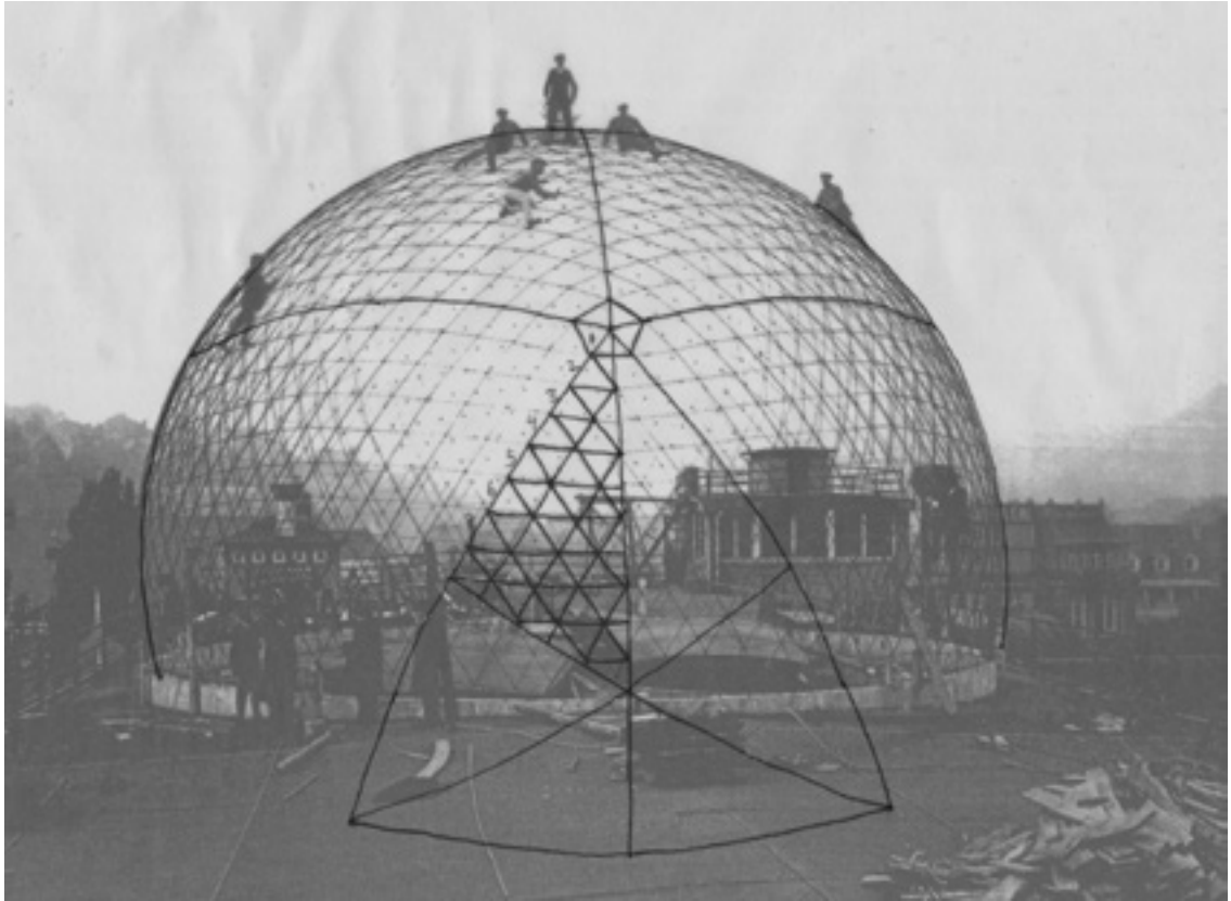
22. Sketch showing the division of the Characteristic Triangle of the hemispherical dome made by Walther Bauersfeld in 1922
