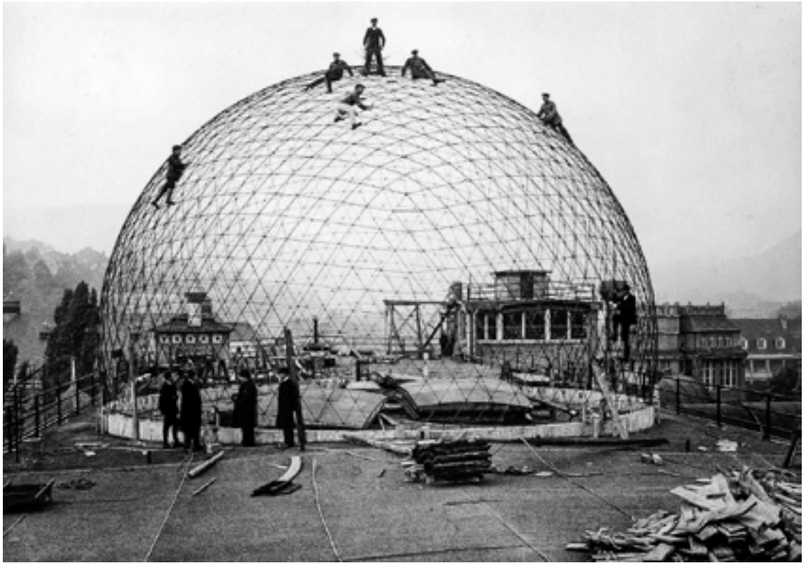
1. Walther Bauersfeld, hemispherical dome using a system of metal bars in Jena, 1922
