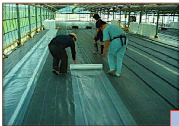
Laying the waterproof sheet
