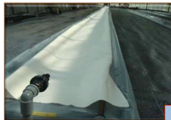
Setting the drip tube of lower side
