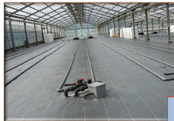
Setting the bed frame with polyvinyl chloride pipes inside a green house
