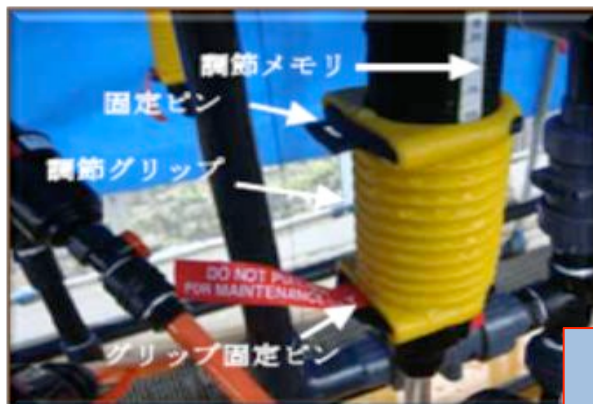
Installing the mixture adjuster
