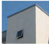
1 CEMENT PLASTER W/ REVEALS & EXPANSION JOINTS
