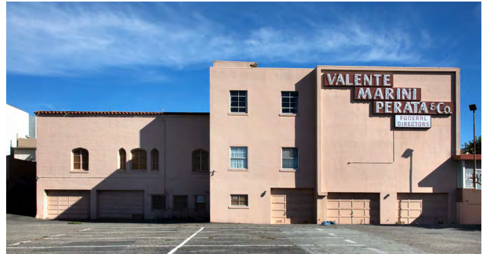
WEST VIEW SHOWS THE ORIGINAL AND 1959 REMODEL COMBINED FACADE
