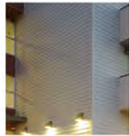
2.1 FIBER CEMENT HORIZONTAL BOARDS 7" EXPOSURE
