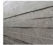
4.1 BOARD FORMED CONCRETE
