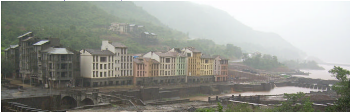
PORTOFINO APARTMENTS (UNDER CONSTRUCTION)
