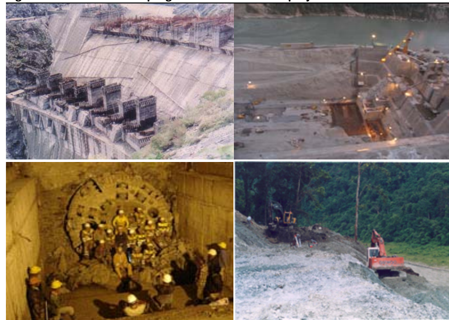
Figure 3: Construction in progress at various NHPC projects
