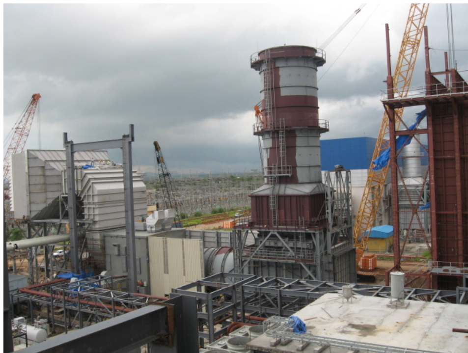
Fig. 1: Gas turbine exhaust
