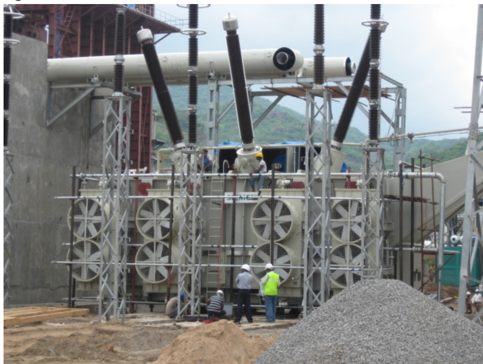
Fig. 2: Gas turbine transformer
