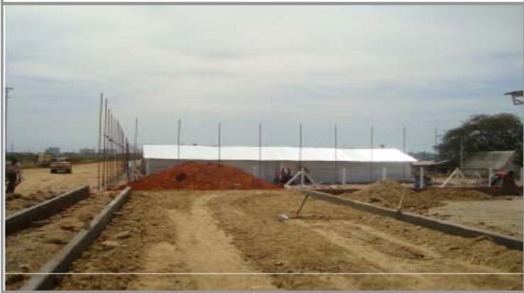
Chennai - Site work under progress
