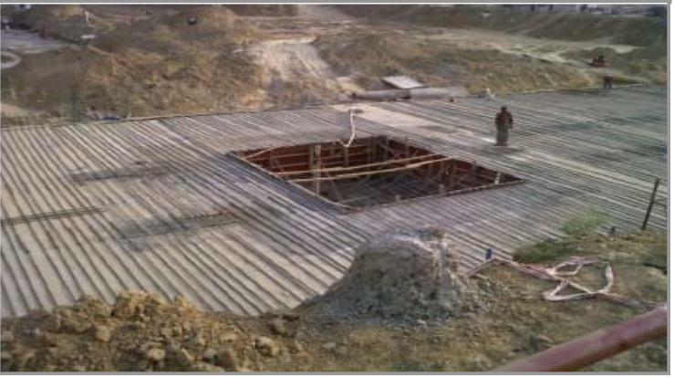
Gurgaon - Ground floor slab work under progress
