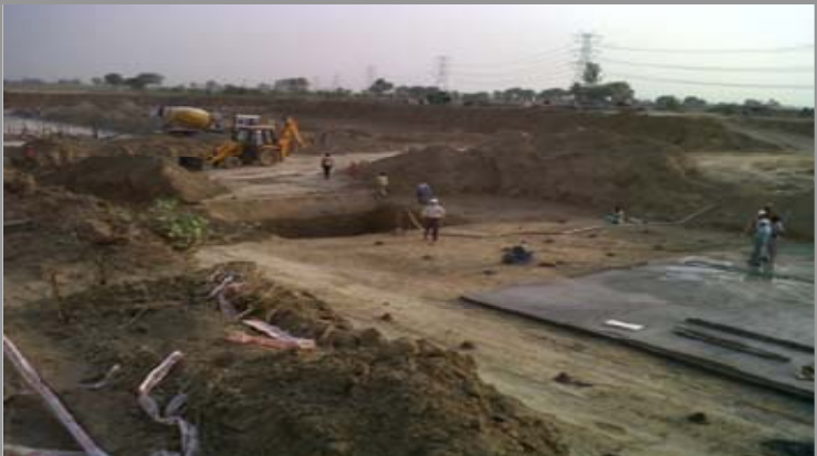
Gurgaon - Excavation and site preparation for towers under progress
