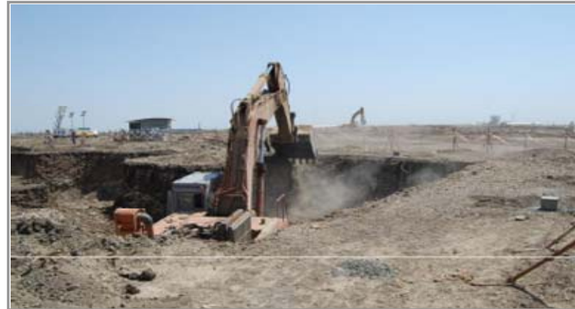
Nashik - Boiler Unit Excavation
