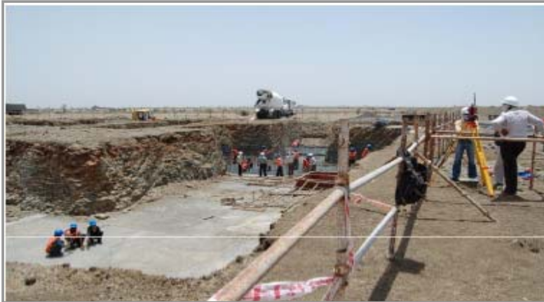
Amravati - PCC & Reinforcement Work in Boiler Unit 1
