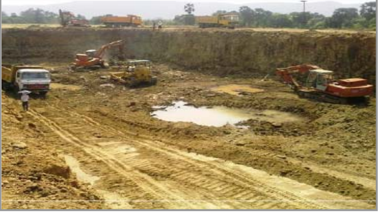
Panvel - Basement excavation work under progress
