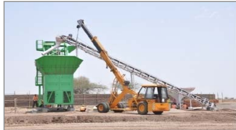
Nashik - Batching Plant being erected
