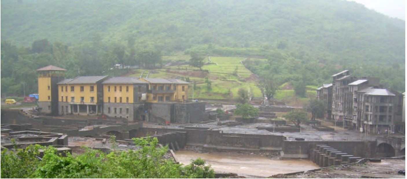
TOWN HALL (LEFT) AND ITC HOTEL (RIGHT) UNDER CONSTRUCTION
