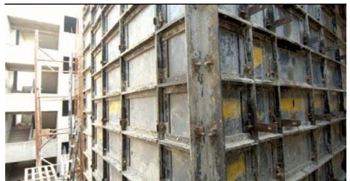
Figure 6: Formwork used for monolithic construction—plastic sheets and steel support
