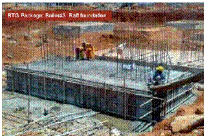
PROGRESS AT THE UTKAL PROJECT
