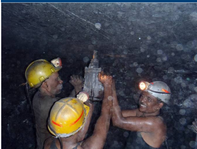
Balgi 1: bore hole drilling under way
