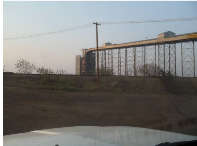
Dipka: coal travels from the hopper to the silo
