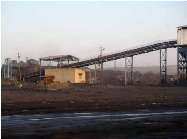
Dipka: conveyors leading to the silo
