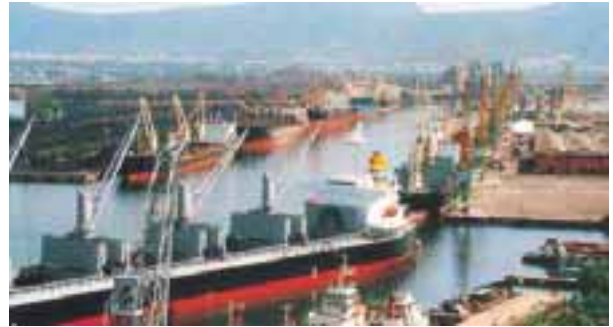
The JNPT port where the capacity will be over 3 million TEU by 2006
