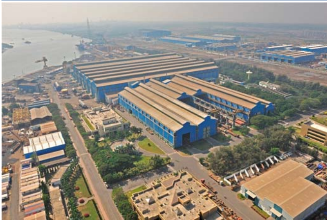
Exhibit 1: L&T – Hazira Complex with new BTG facility along side old fabrication yard
