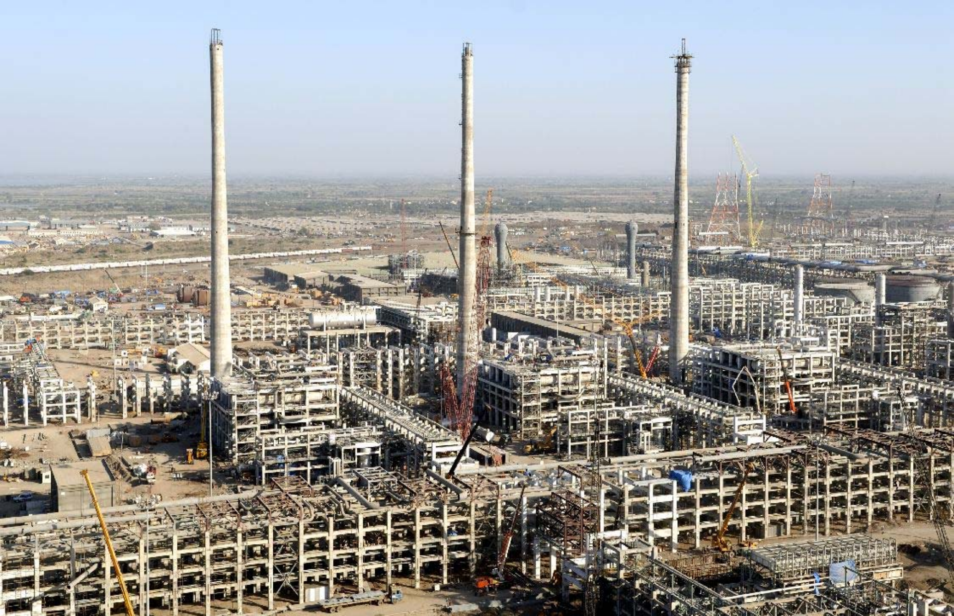
Overview of the Sulphur Complex
