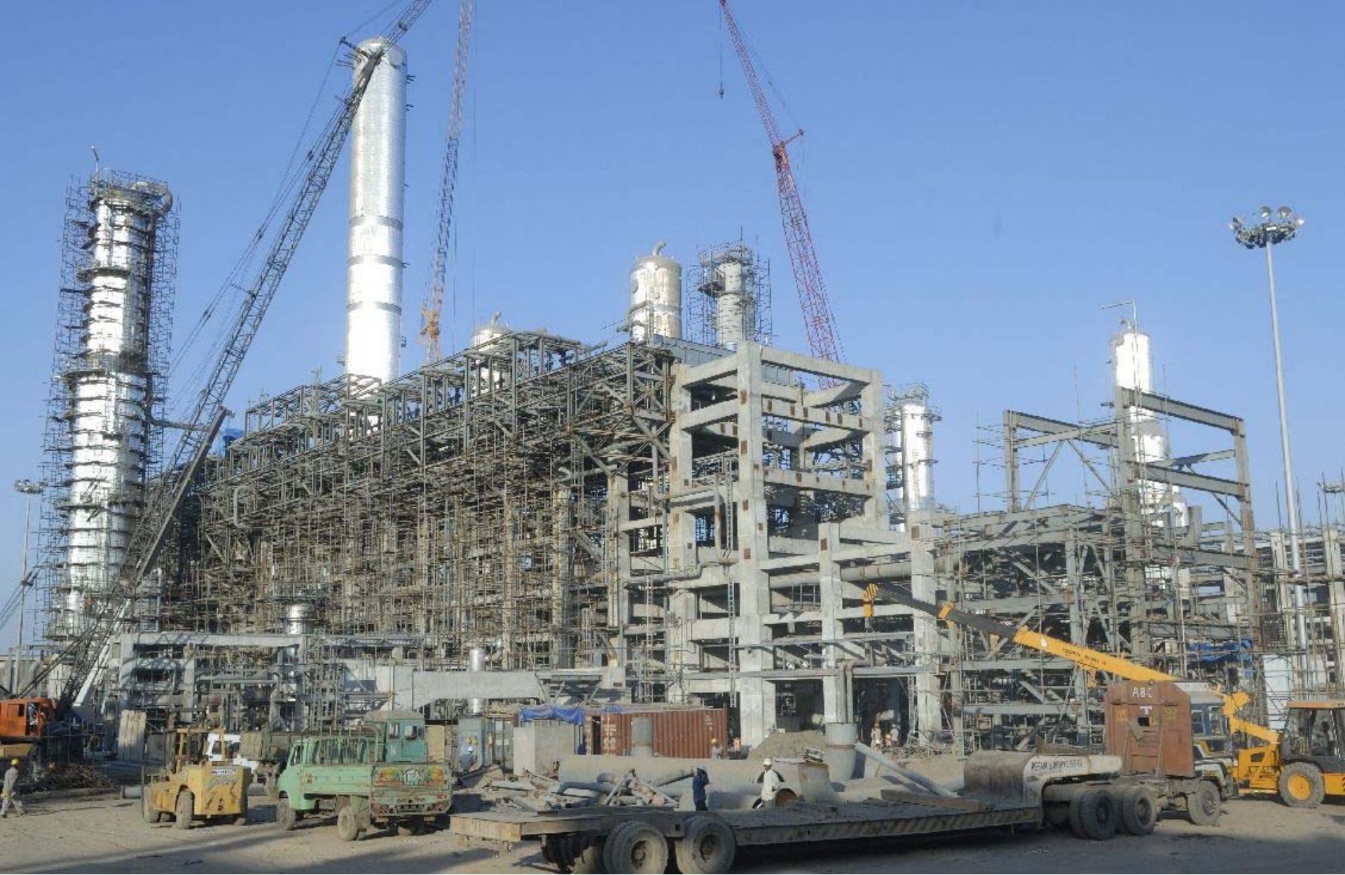
Propylene Recovery Unit (PRU) installation nearing completion
