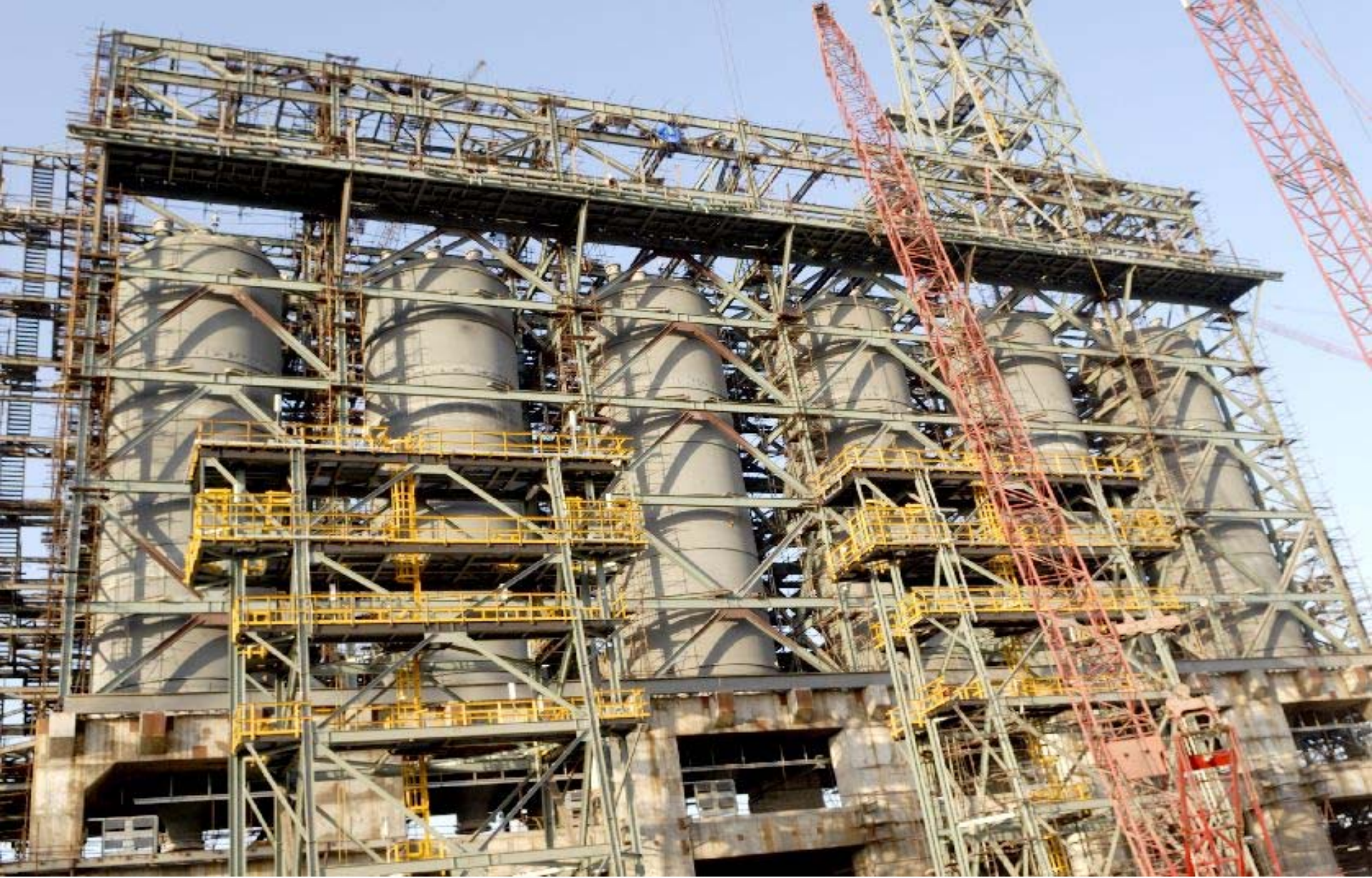
Installation of 6 Drum Coker Structure nearing completion
