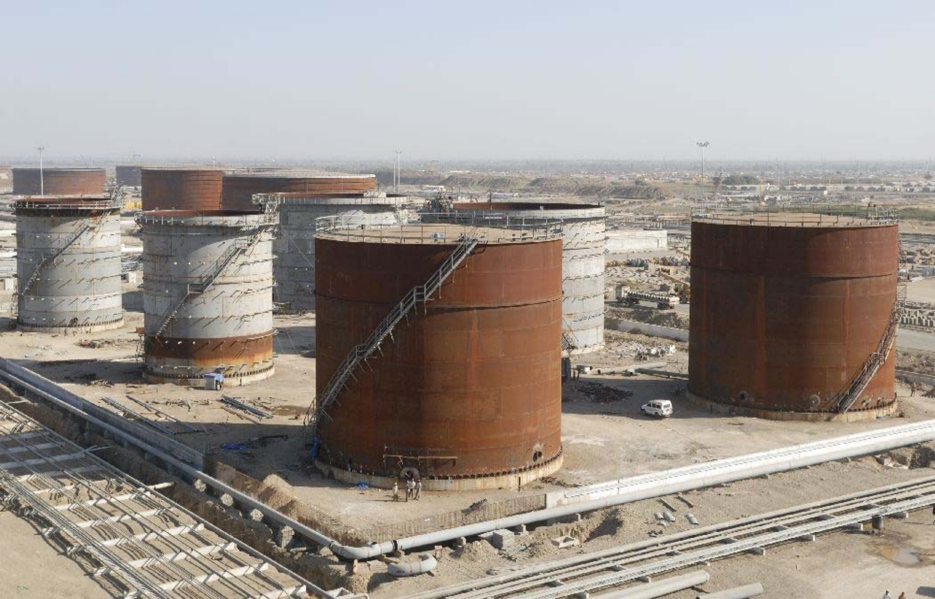
Overview of the Refinery Tank Farm
