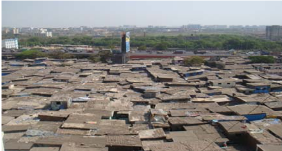
Exhibit 2 Golibar Project Site (facing Western Expressway)
