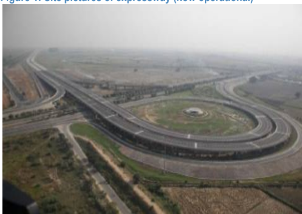
Figure 1: Site pictures of expressway (now operational)
