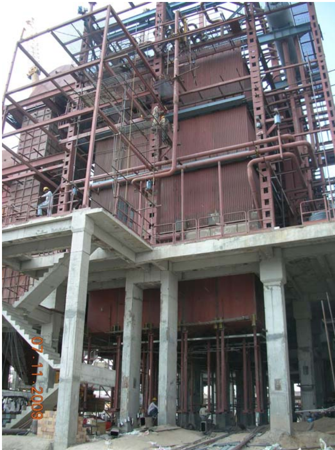
Fig 6 - Construction work in full swing...
