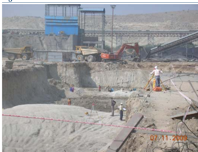
Fig 3 - Unit 8 construction site in Ras
