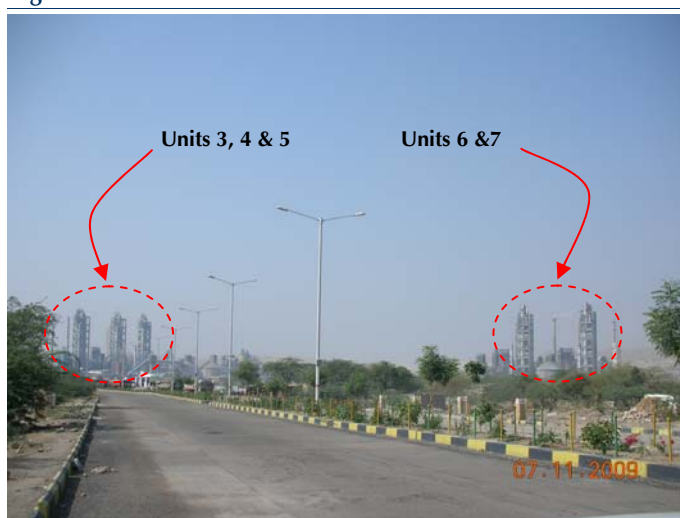
Fig 2 - Five cement units in Ras
