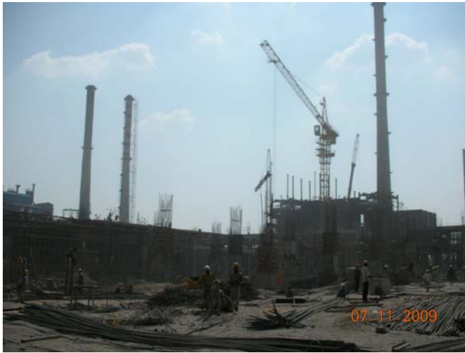
Fig 4 - 100MW power plant site...
