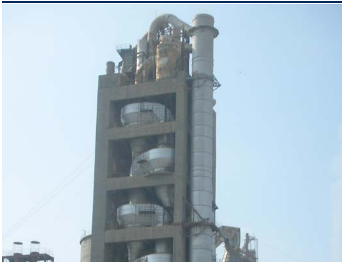
Fig 11 - Piro process – Pre-heater
