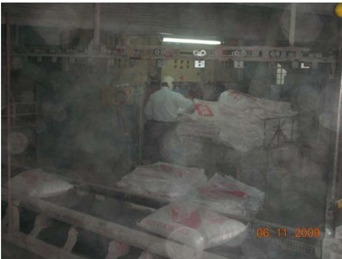
Fig 15 - Cement packaging unit
