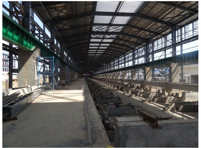
Fig. 4: Smelter under construction
