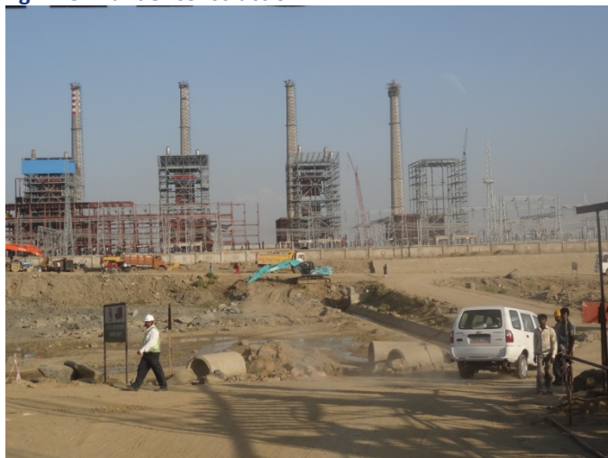
Fig. 1: CPP under construction
