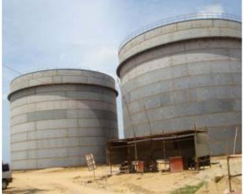
There are two UF product and Backwash tanks with volume of 13800 cubic meters each. This process is primarily used in cleaning Reverse Osmosis (RO) membrane filters. It would enable to increase the life of RO membrane up to 5 years as against normal life of 3 years.
