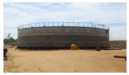
The desalinated distilled water gets stored in this tank before it goes to the next stage of minerlisation to make it potable.
