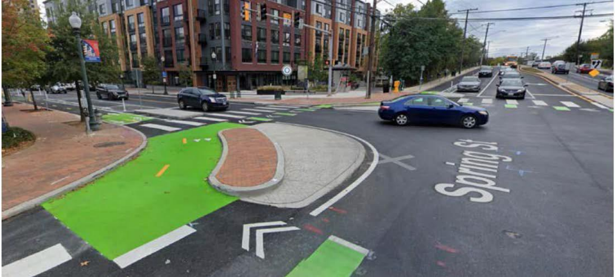
Figure 4. Truck apron and protected intersection in Montgomery County, MD
