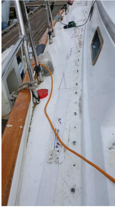
Port side templates drilled and bolted.
