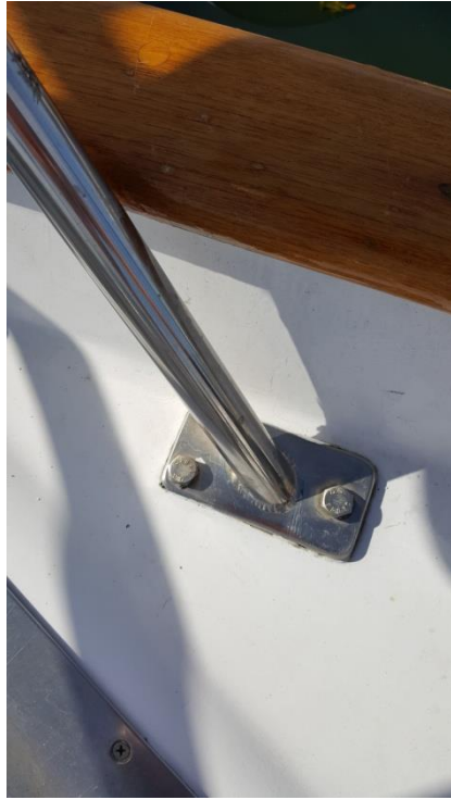
Other sites for anti-leak blocks... Aft rail mounts!
