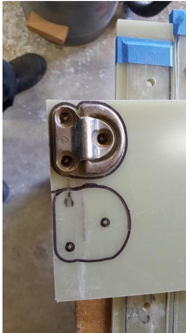
Tracing Running Back Stay & Jack-line Folding Pad eye blocks
