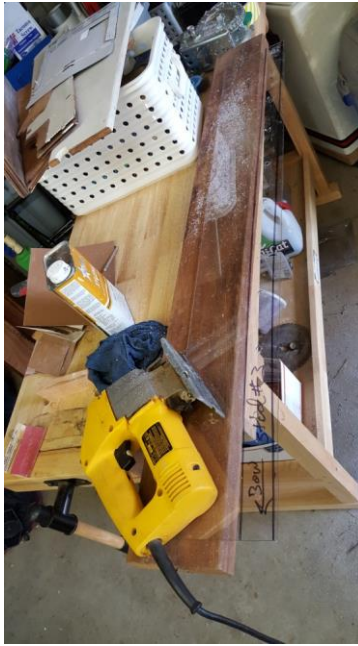
Step 5: Cutting out Makrolon with jigsaw
