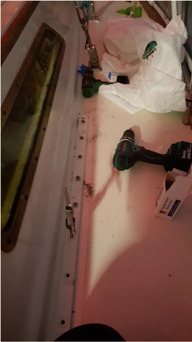
The Home stretch... Drilling/Re-Tapping out holes to chase out captured internal threads below deck.
