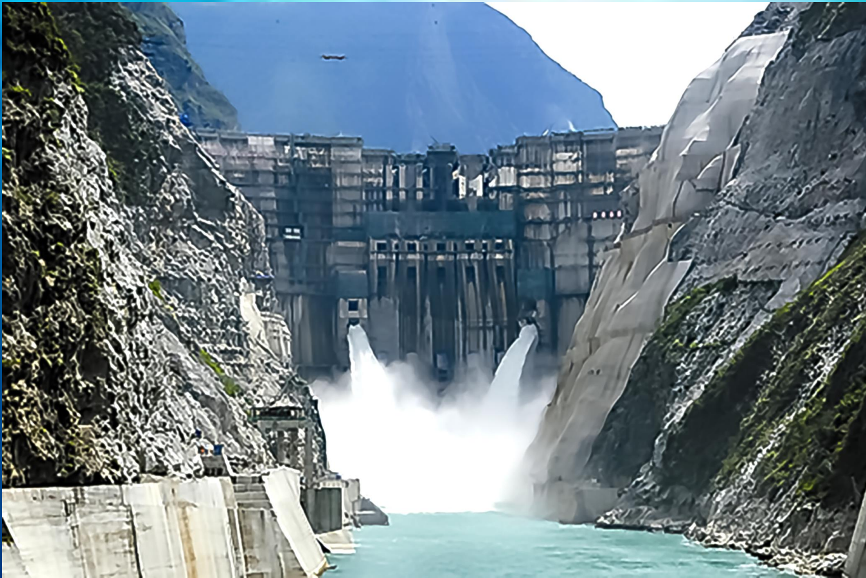
The tallest dam in the world at 305 meters is the Jinping dam on the Yalong river in China.
