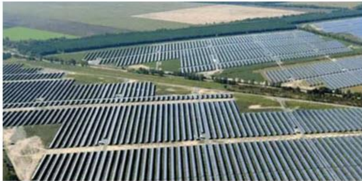
16,000 square meters per megawatt
