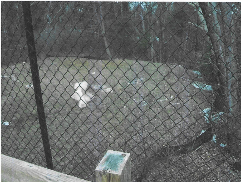
Erosion controls observed throughout the site, should be removed
